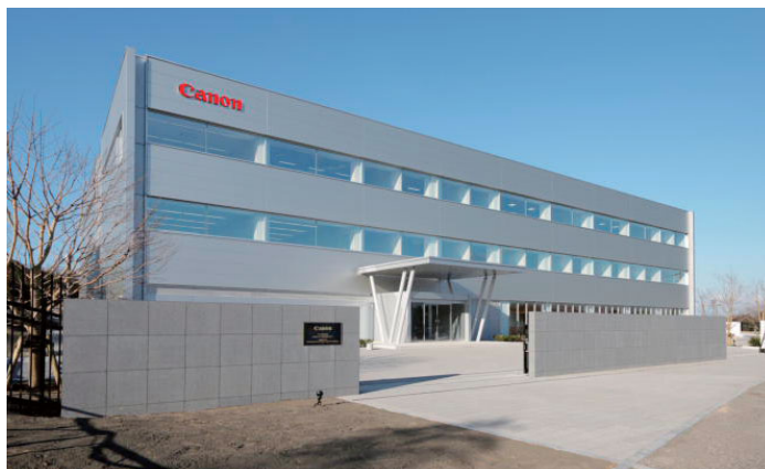
Production skills training facilities in Oita
