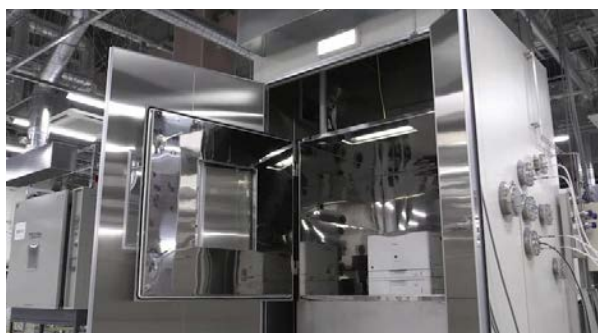
Chemical emission evaluation testing laboratory
